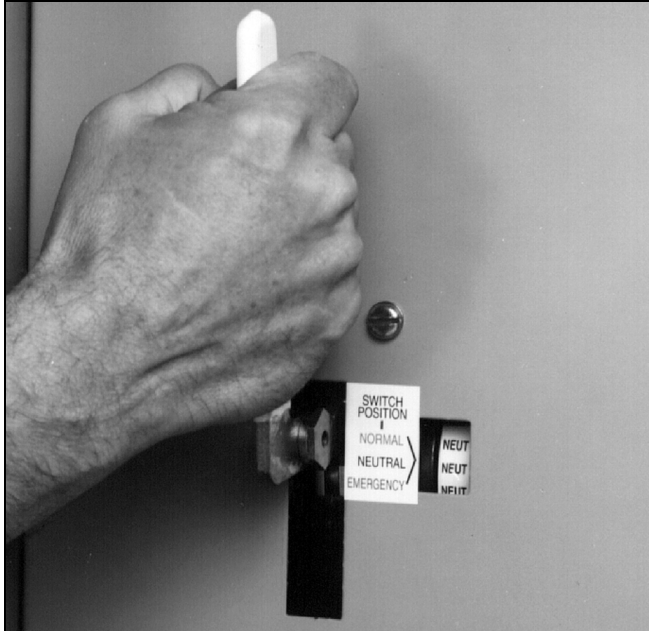
Figure 32.ATS Manual Operating Handle in Use (225-1200 A Models).
