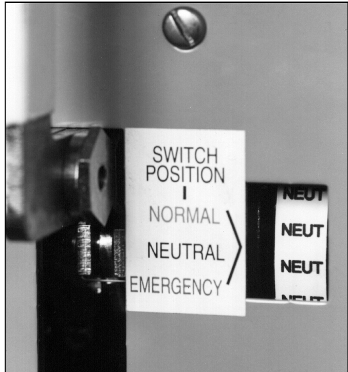
Figure 34.Indicator Wheel in Neutral Position (225-1200 A Models).
