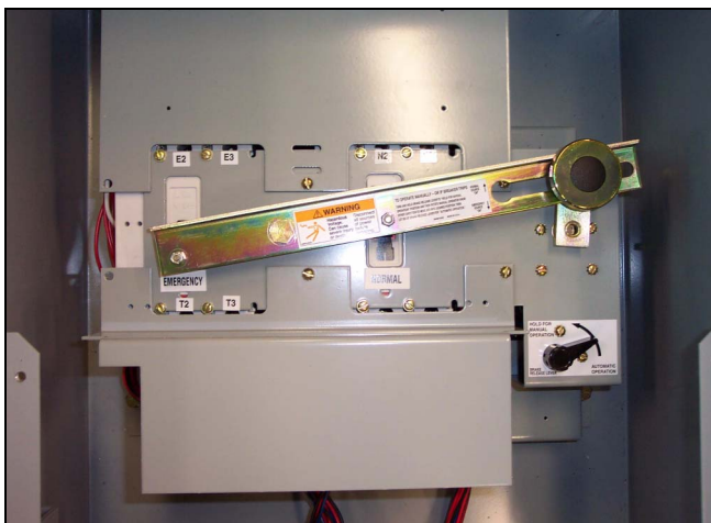
Figure 8. Typical Power Panel for 30-150 A Models.
