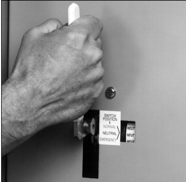
Figure 32.ATS Manual Operating Handle in Use (225-1200 A Models).
