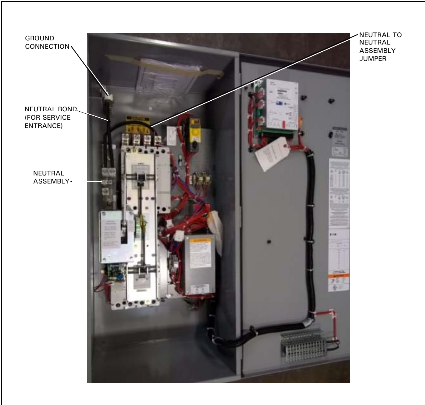
Figure 19A. 4 Pole Neutral Bond for Service Entrance
